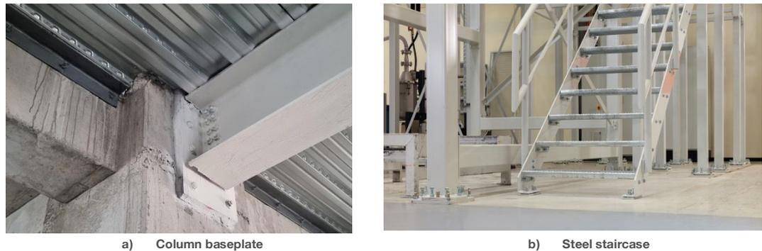
Fig. 7.1: Examples of primary and secondary connections
